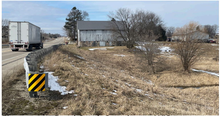
Figure 2.02 - Dead Creek Crossing on WIS 60
