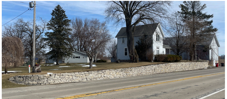
Figure 2.03 - Retaining Wall on WIS 60
